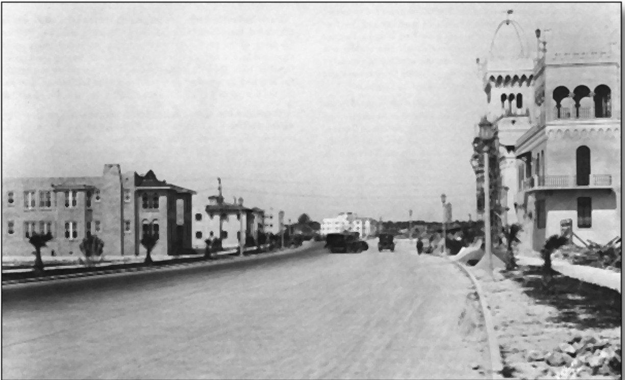
CONSTRUCTION CONTINUES ON BOOM-TIME DAVIS ISLANDS
