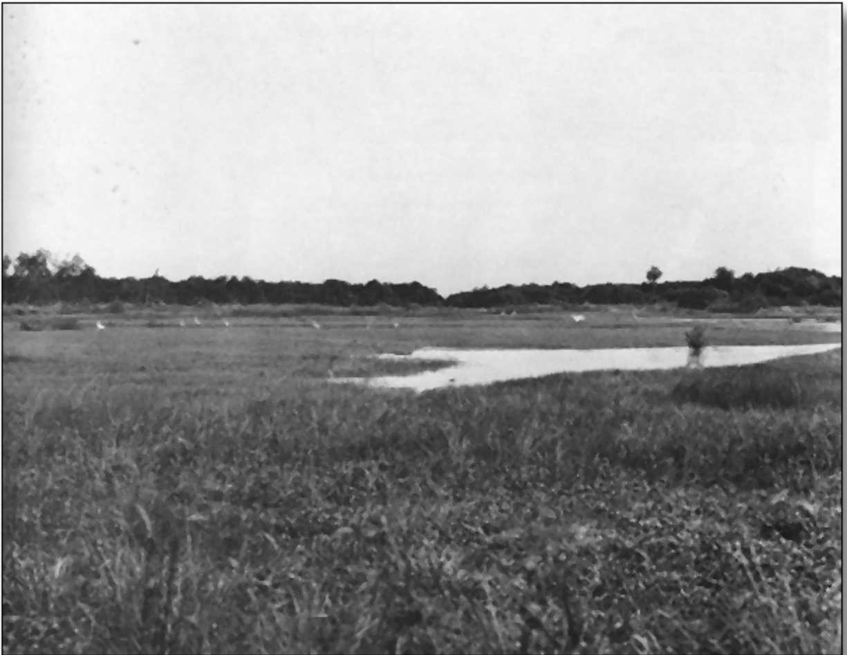
THIS MARSHY SCENE soon gave way to the bulldozers and carpenters as Davis Islands was dredged up. This view was made in 1924.
